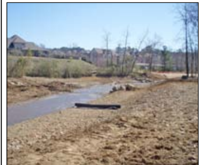
The banks have been graded and will be planted with native plants.
