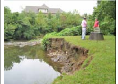
Above: Little Shades Creek before construction: Vertical, undercut banks.
