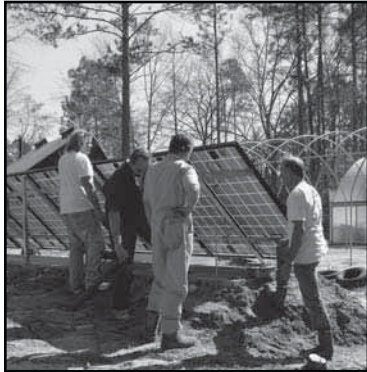
SOLAR GREENHOUSE installation of solar panels
